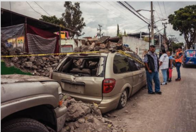
Photo of devastation to buildings/roads caused by a recent high-magnitude earthquake, e.g. Mexico 2017
